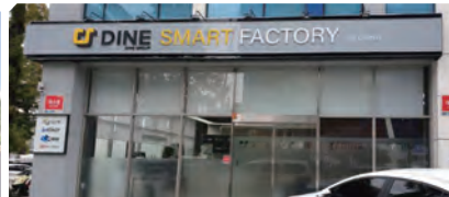
Nambu Support Center(SMART FACTORY)
